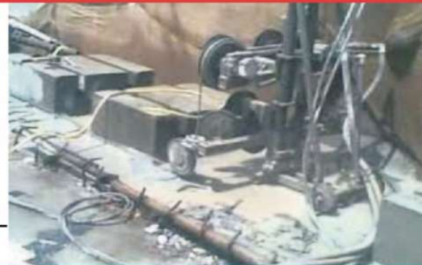
Sugar Factory foundation cutting work
