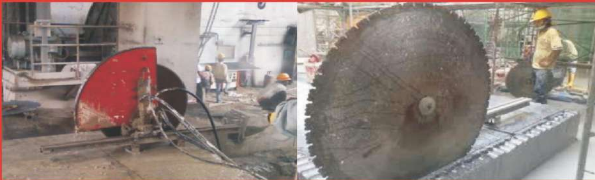
→ RCC foundation cutting work
