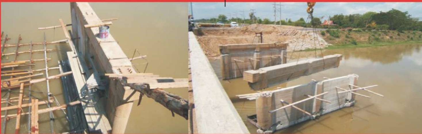
RCC Heavy Bridge Cutting Work
