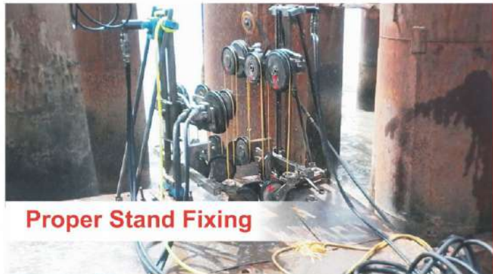
Diamond wire seating on cut out Location
