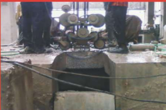
RCC foundation after cutting
