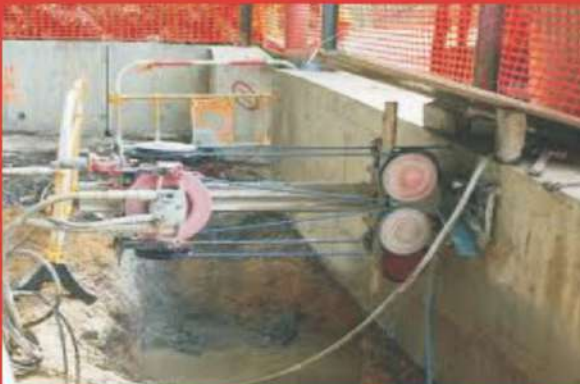
RCC Compound wall cutting work
