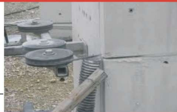
RCC Column cutting work
