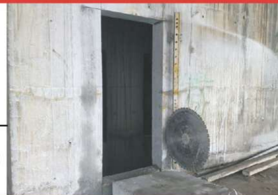
→ RCC Wall After Cutting
