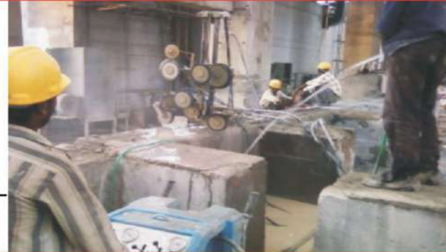
Cement plant foundation cutting work
