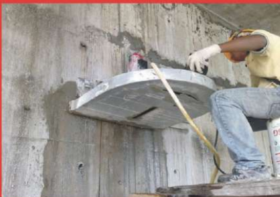
→ RCC Wall Cutting work
