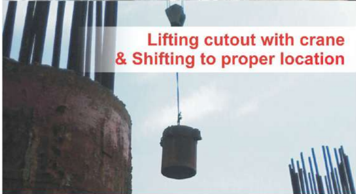
Pile after cutting
