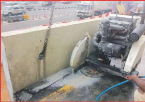
RCC Slab cutting work
